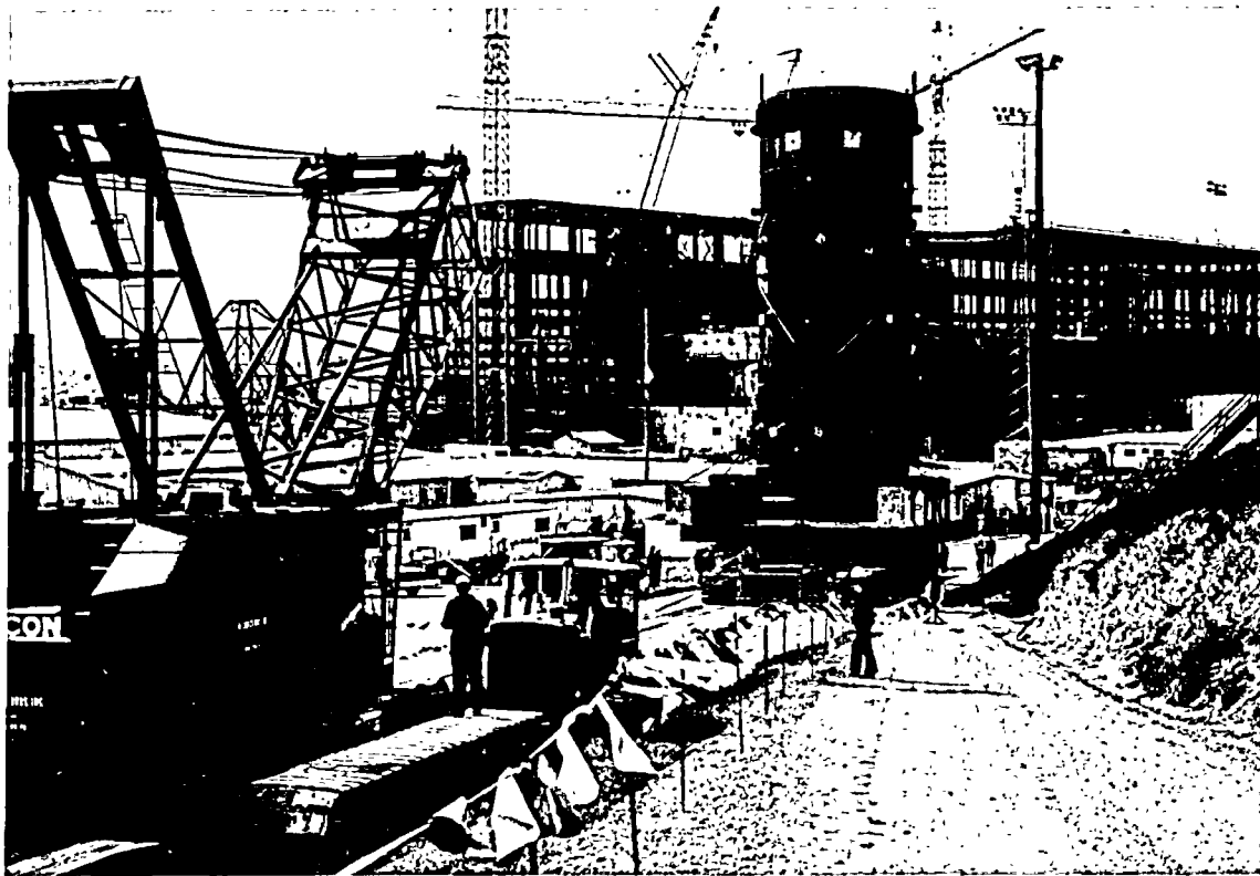
The reactor pressure vessel for Limerick Generating Station Unit 1 near Pottstown, Pa., is moved down a hill to a place where it will be installed in the reactor containment. The 1100-ton vessel inched along as an NRC inspector (in white helmet, below vessel) checks on its progress.
